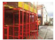
Insert the POSTS - hooks facing the boards & adjust if required Post knuckle is the same height as the board support. Hang the SOLID PANELS with the CONCAVE baseplate facing the boards and if required use the Hop up and short board to aid your height.
