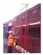
Access Points usually located at the ends of the runs or away from the main work location. Using 2-POSTS, insert the LADDER RESTRAINT Using 2-men – CAREFULLY raise the 2-POSTS in unison and lower into the STABILISERS and locate your pins to the desired height. OR: Use an adjacent Set of Staybills MEDIUM to work off.
