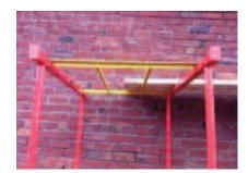
H-FRAMES are placed between Staybills to provide additional Board support - The H-frames in can eliminate trip hazards and provide a smooth platform when working in 10' or 13' Board lengths in Bay 4 or 5 respectively.
