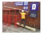
If the platform is adjusted too high for the user's height, rest 2-short boards on the lower transom to aid the placing of the 3-scaffold boards to form your platform. Hop up boards sitting on the lowest transom with 3-short boards resting to form easy access & additional height.
