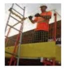
Insert the LADDER & secure to the LADDER RESTRAINT. Only access the platform when ALL Solid Panels have been erected. Option: Use C-HOOK upside down on the POST to support the Gate forming Solid Panel and finally, hang the Orange Large panel at the return.
