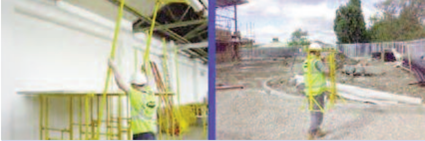
Left Photo shows Ladder Restraint inserted into 2-Posts for higher platform levels to remain safely on the ground.
